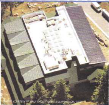
PHOTO COURTESY OF OPEN ENERGY CORP., SOLANO BEACH, CALIF.
