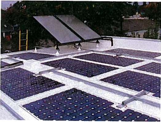
Sweet Life Pâtisserie's retail store in Eugene, Ore., features an Open Energy 10.8-kW SolarSave system and a solar water-heating system comprising two SunEarth EC-32 collectors. The tree in the background of this photo has been removed to eliminate shading on the panels.
